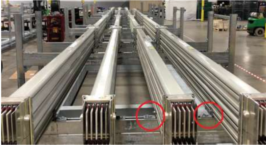
Al Housing has grooves both side Slide T Bolts Fix
